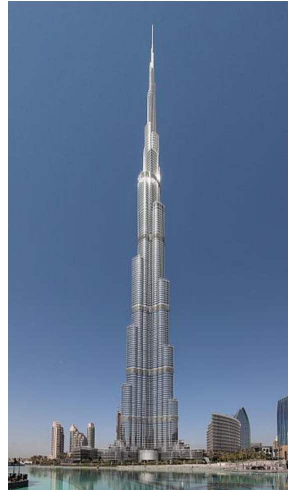
Burj Khalifa, the tallest building in the world (Photo use permission granted under GNU Free Documentation License)
